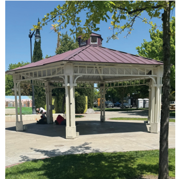
Shade structure surrounded by tiered seat walls at Library Park.
