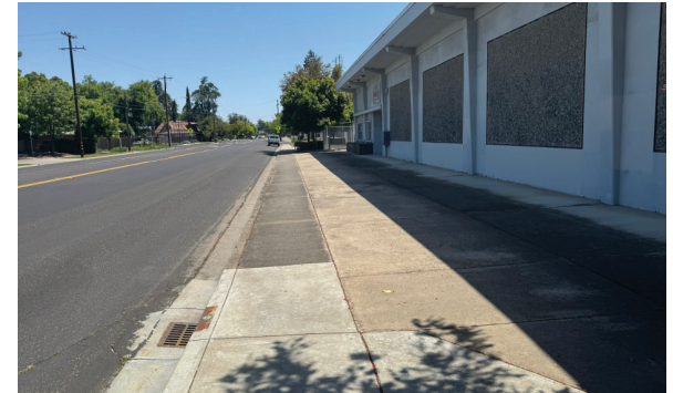
Paved frontages along W. Center St.
