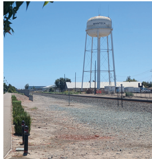
View of rail corridor and water tower today.
