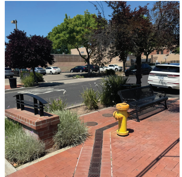
Brick paving, trench drains, metal, and brick identity markers, and seating at bulb-outs in the Downtown Core.
