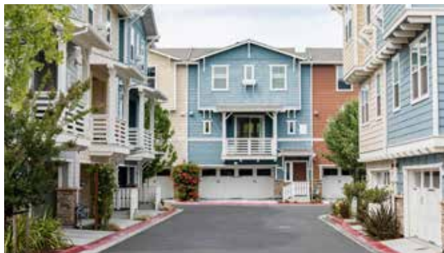
Individual garage doors facing each other.
