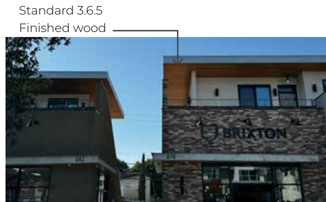
Examples of architectural detailing, materials, and color.
