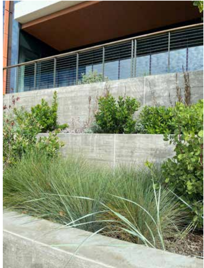
Landscaping above a retaining wall, as described in Standard 5.3.3(C).
